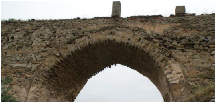
Fig. 5. Building the arch in the Roman method in one of the spans
