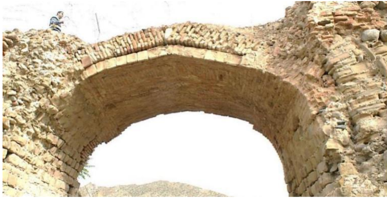
Fig. 4. Building the arch in the form of archivolt with bricks and combined
